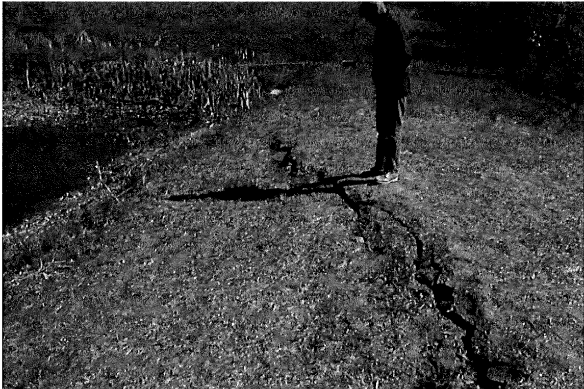
Longitudinal crack.
