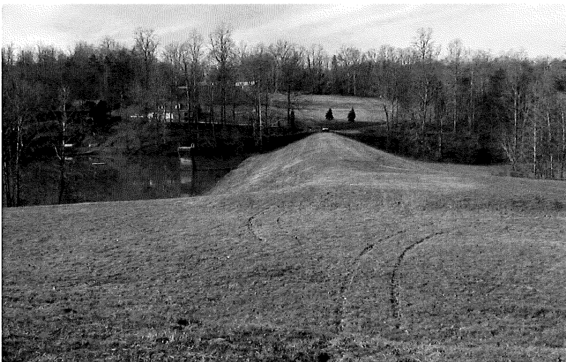
Left: A vegetated earth spillway.
