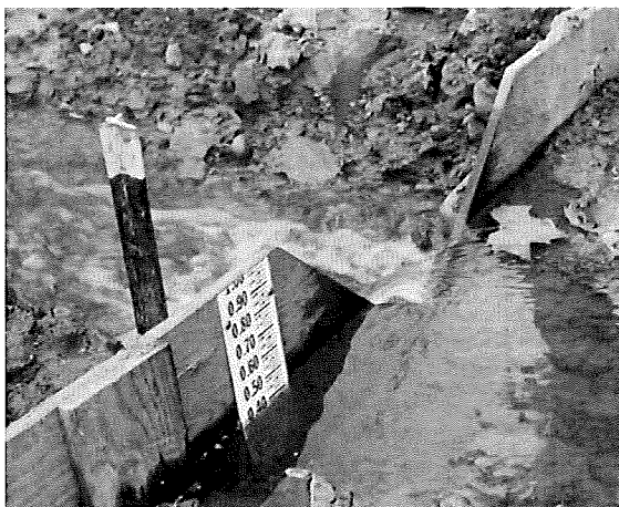
Right: V-notch weir Used to measure seepage.
