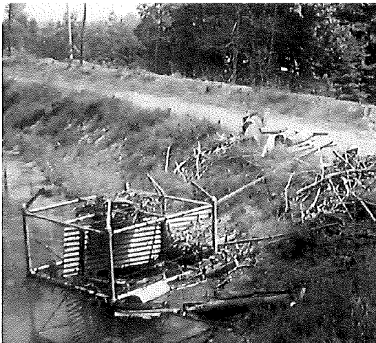
Far right: A damaged trashrack caused by the hammering forces of debris.
