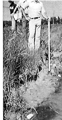
Left: Beaching of an upstream slope.
