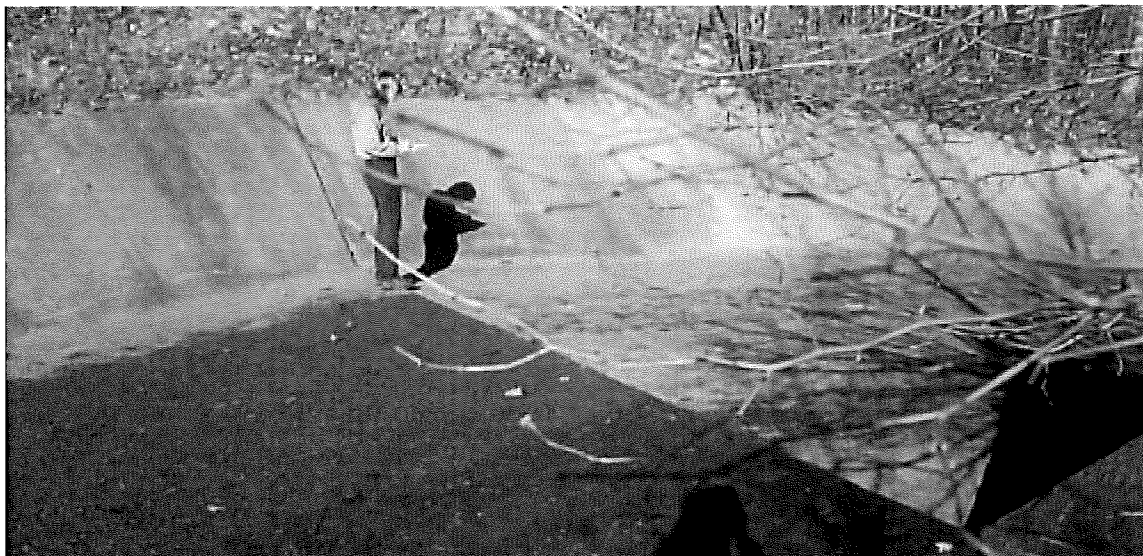
Flow entering the joint of a spillway floor slab.
